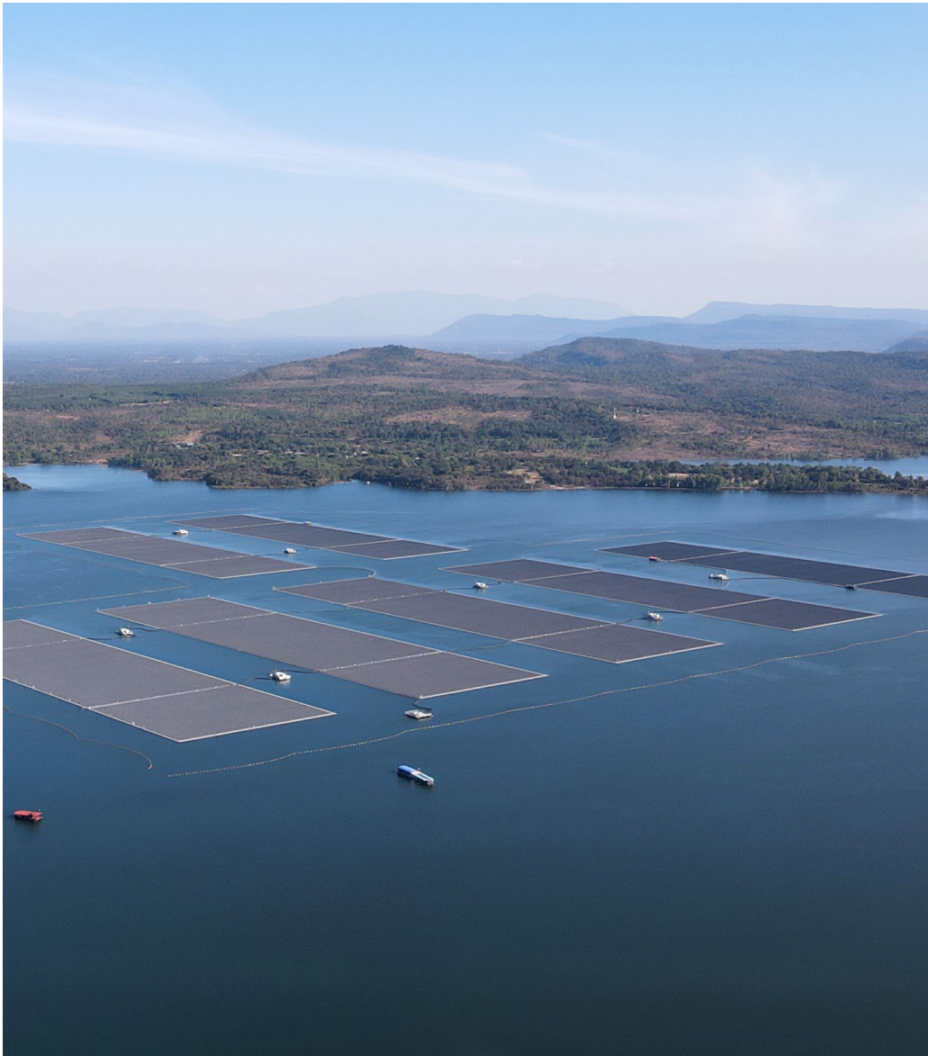
Sirindhorn Dam Hybrid Solar-floating Project
