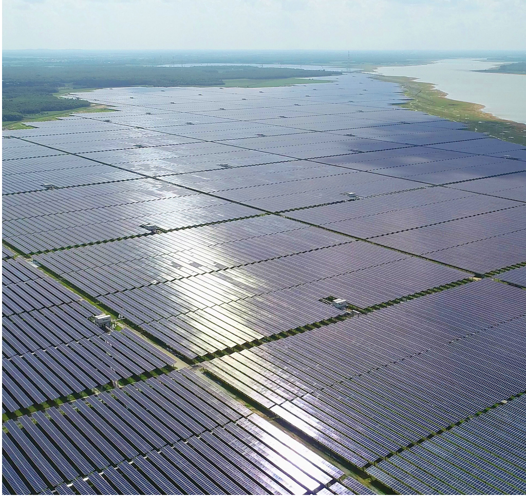
Dau Tieng Solar Power Project, Vietnam
